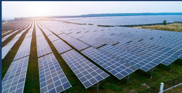
The project activity is a solar power project with a total capacity of 10 MW implemented in Halagaladdi, Hiriyur taluk, Chitradurga district, Karnataka, India. The electricity (16,623 MWh/year) generated from the project activity is supplied to the Bangalore Electricity Supply Company Limited (BESCOM).
